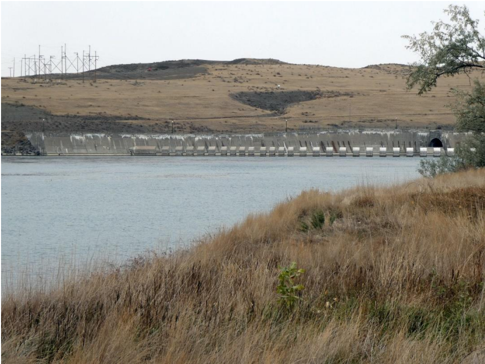
Below the dam near the powerhouses
