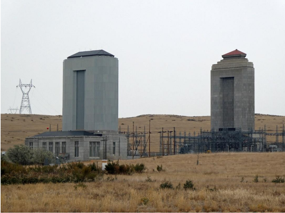
The powerhouses at Fort Peck Dam
