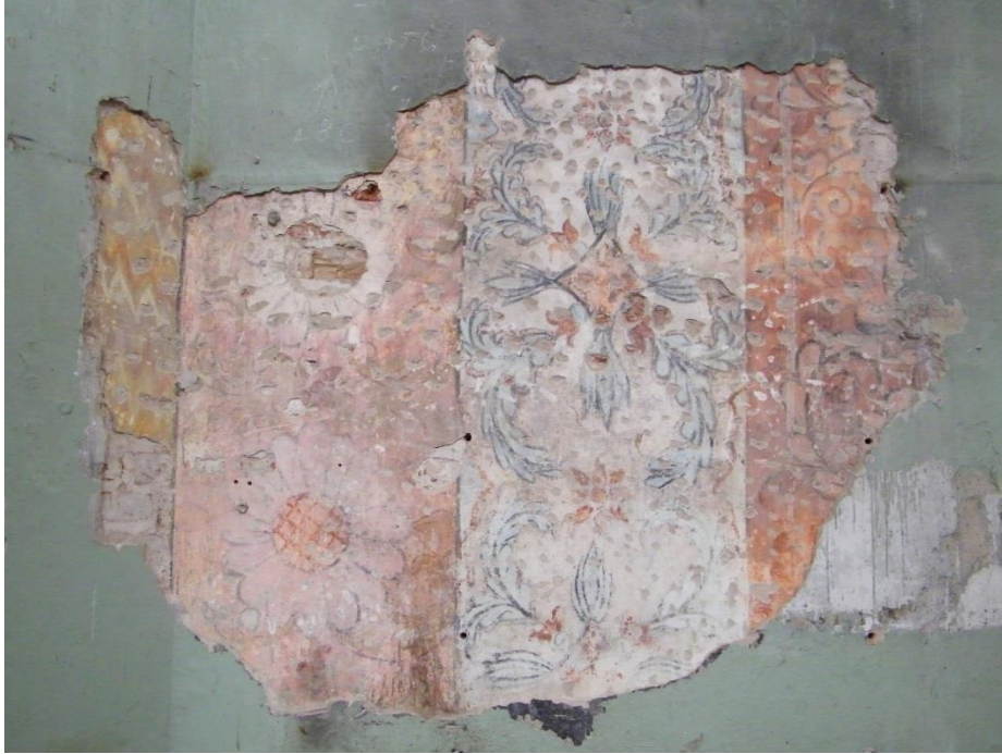
Old frescos had been plastered over in the Church of the Holy Trinity.
