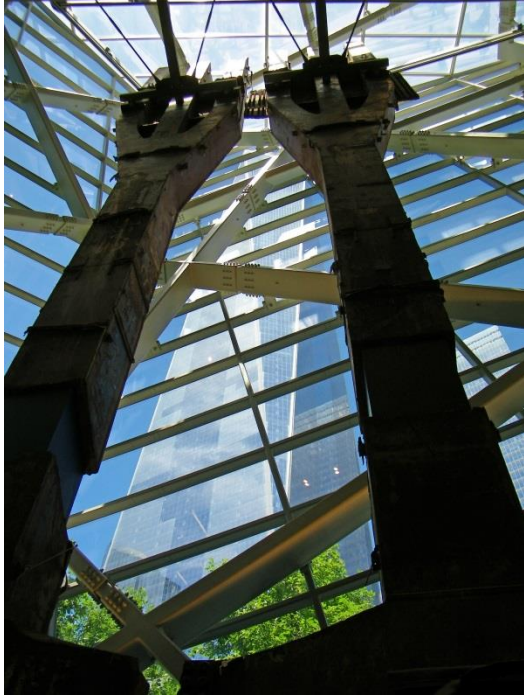
Remnants of the original World Trade Center frame the new Freedom Tower
