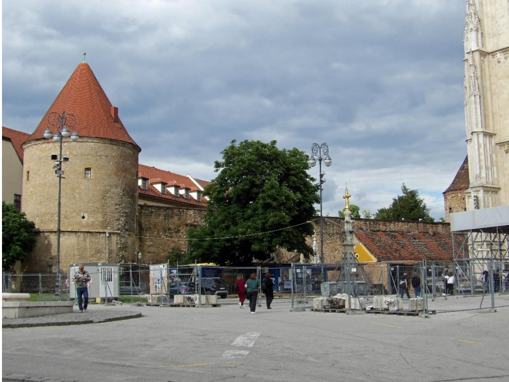
Kaptol's fortifications date back to the 1400s. A surviving segment can be seen next to the cathedral.
