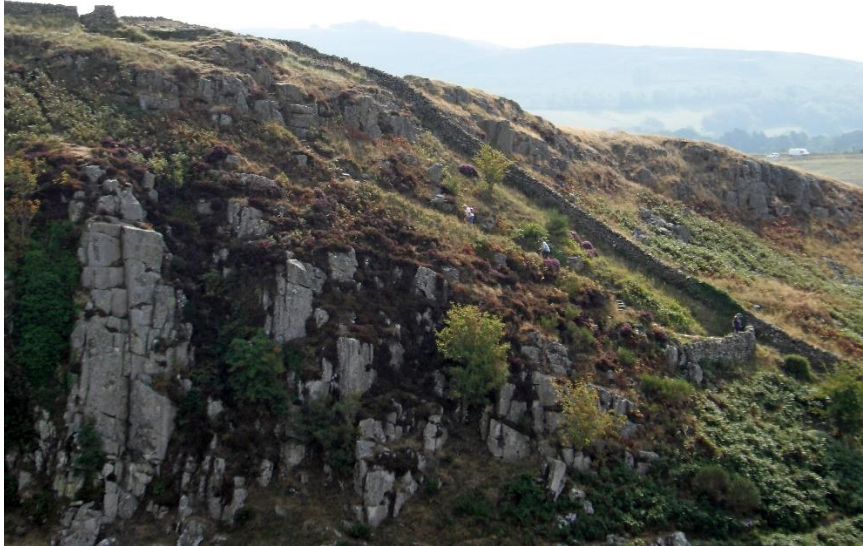
Hadrian's Wall climb Steel Rig in Northumberland National Park
