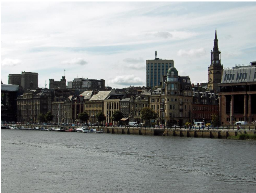
View from Gateshead across the river towards Quayside
