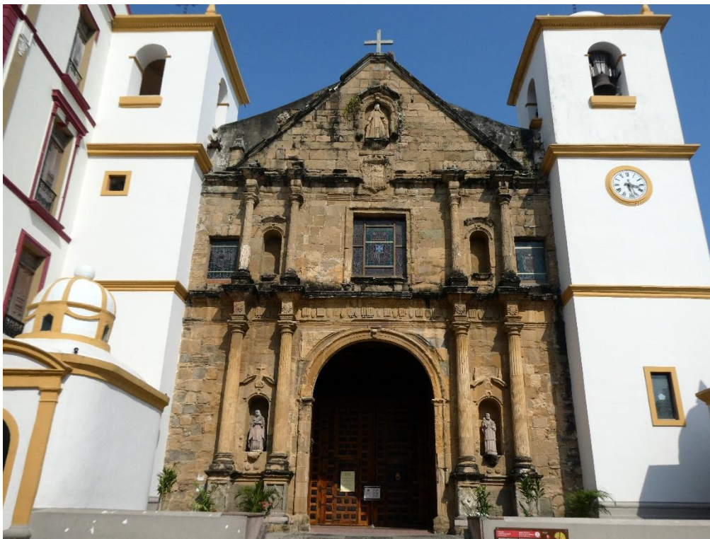
Our Lady of Mercy Church. The baroque stone face of the church was removed from the Convento de la Merced ruins site in Panamá Viejo and reassembled here.
