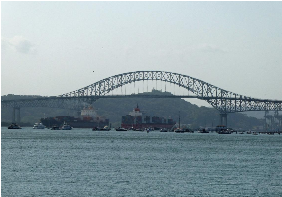
Two cargo ships pass one another beneath the Bridge of the Americas.
