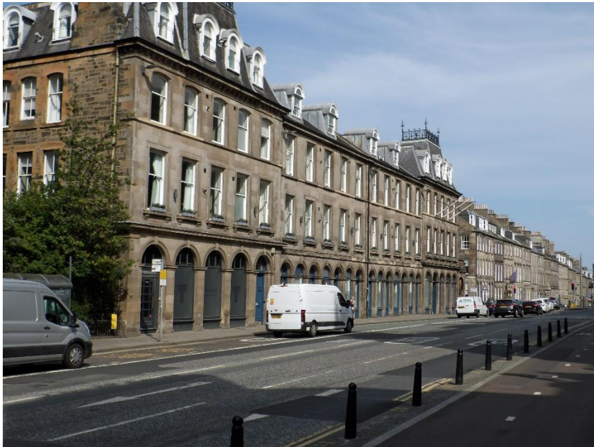
New Town's Queen Street
