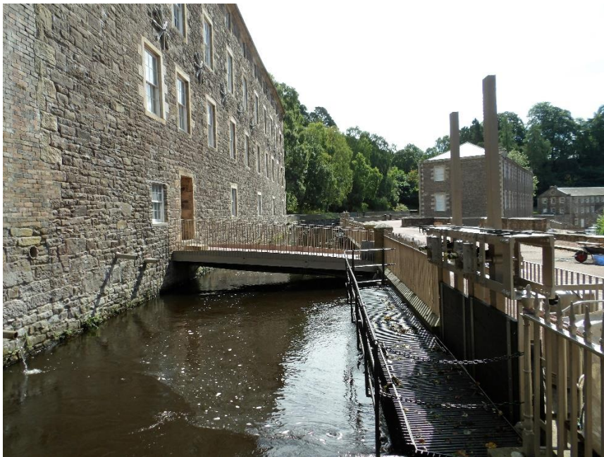
Taking advantage of the elevation of the waterfalls of the upper Clyde, water was diverted to this channel at New Lanark where it then drove waterwheels whose rotation drove the belts connected to the mill buildings that in turn ran the equipment in the buildings that spun cotton into thread and that performed large-scale weaving.
