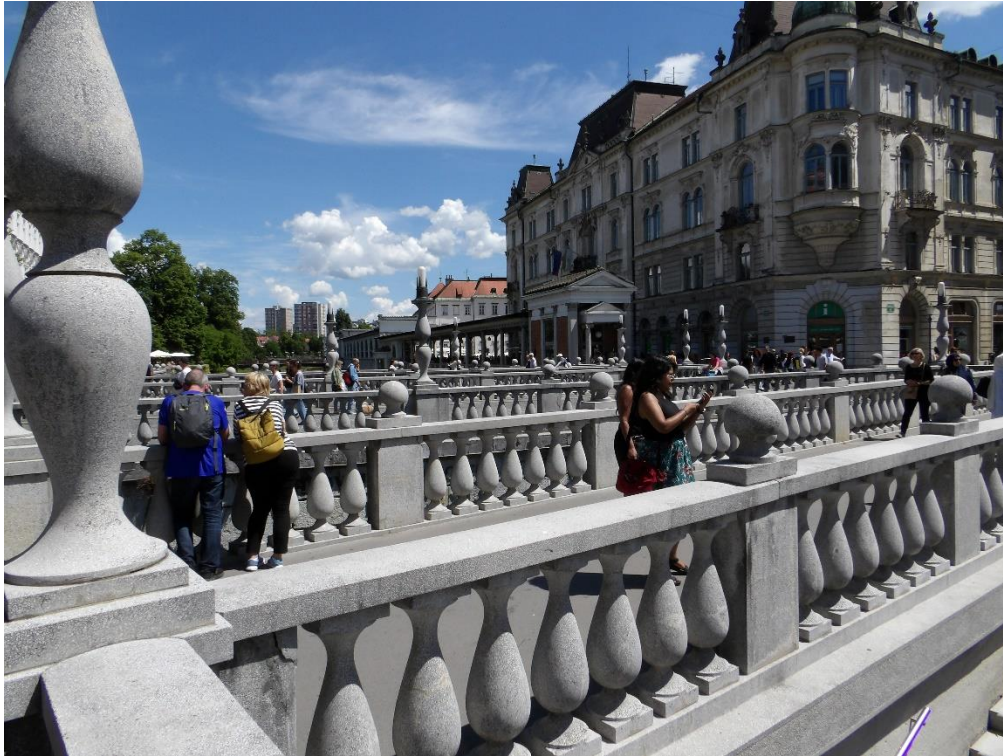
The Triple Bridge. When one historic bridge proved to be too narrow for both vehicles and pedestrians, rather than replace it, two pedestrian bridges were added, one on each side.
